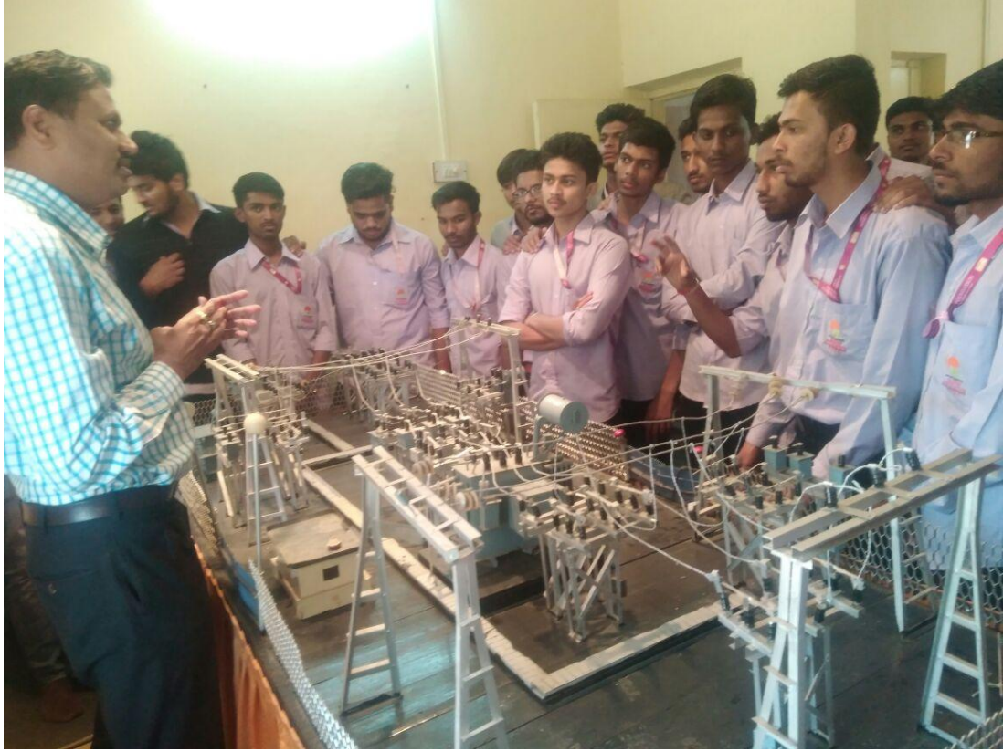
Er.S.Patil illustrating the various equipment used in Substation
