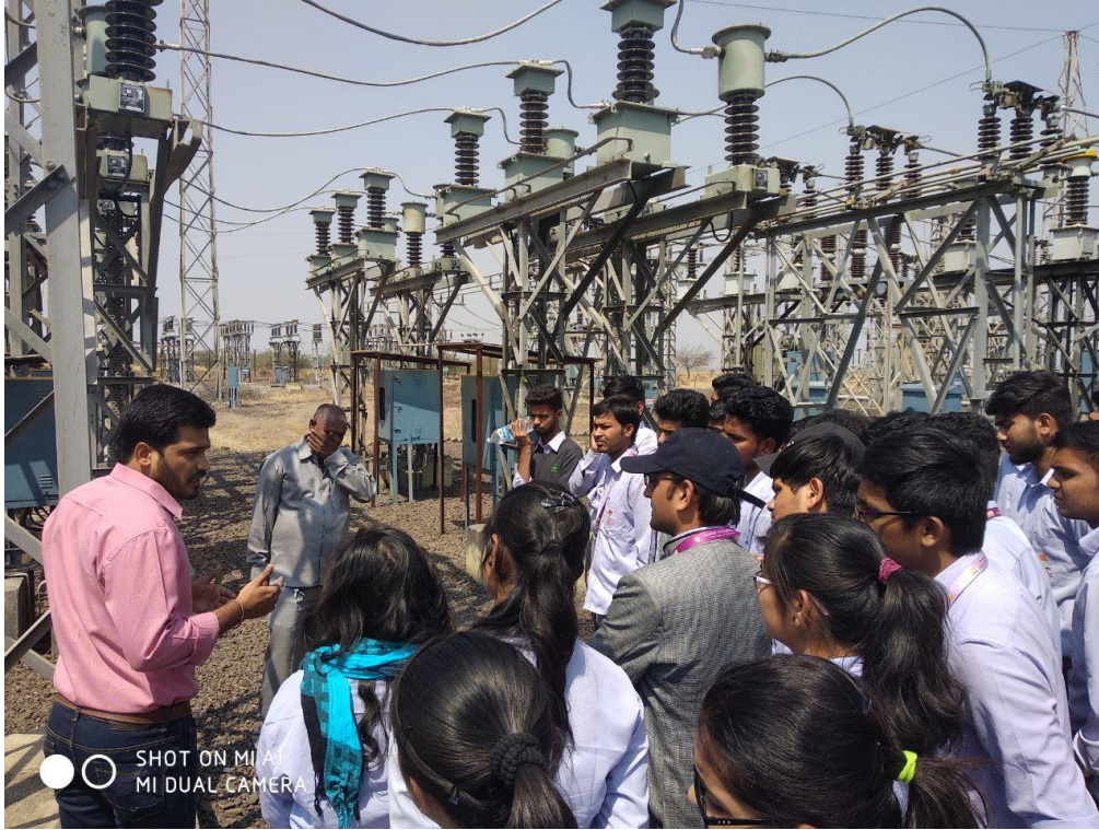
Er. Suarj Patil Explaining substation layout to Students
