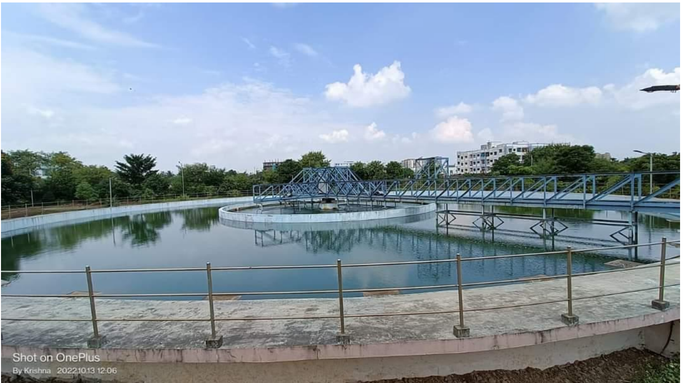
Clariflocculator View at Nilgiribaug WTP
