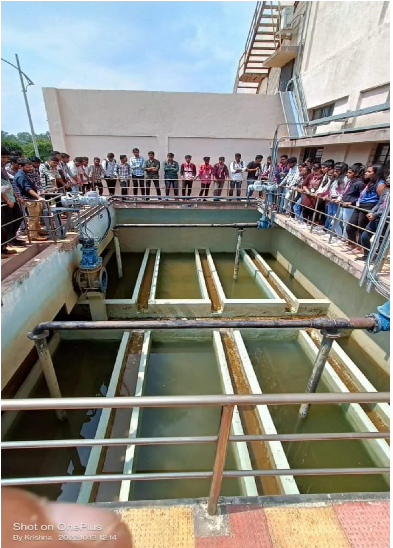
Rapid Sand Filter Under Cleaning (By Backwashing Process)
