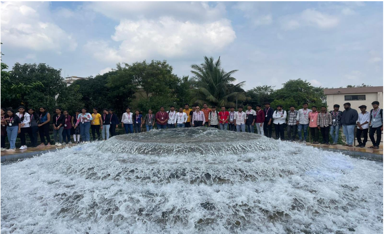
Cascade Aerator View at WTP
