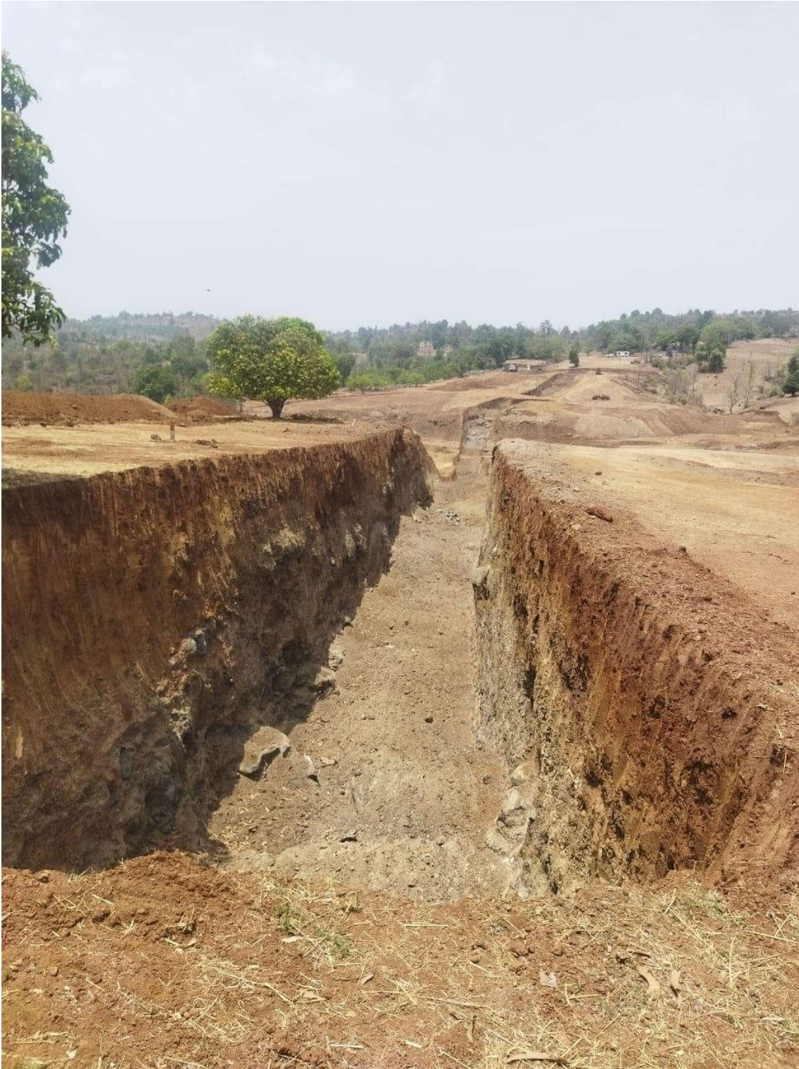
Excavation of COT of Gadavane Earthen Dam
