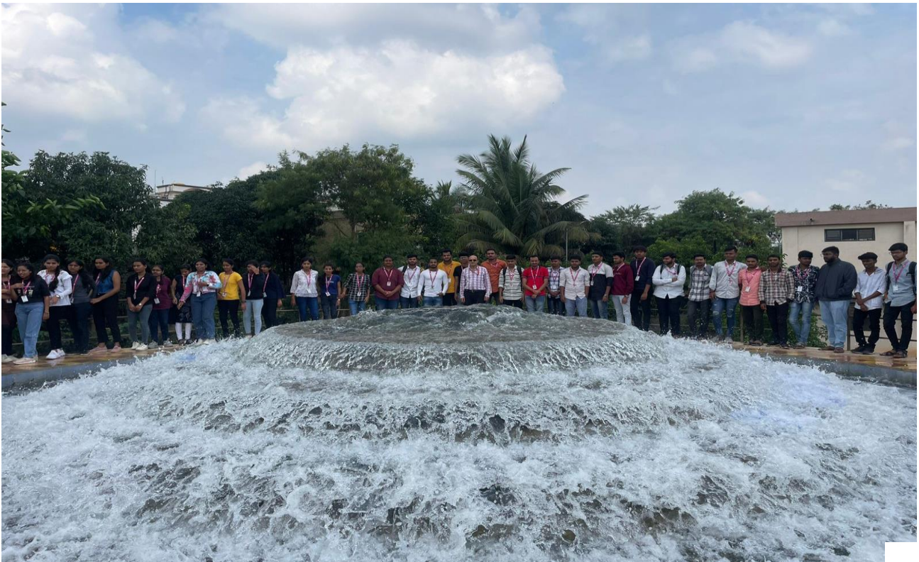
Cascade Aerator View at WTP
