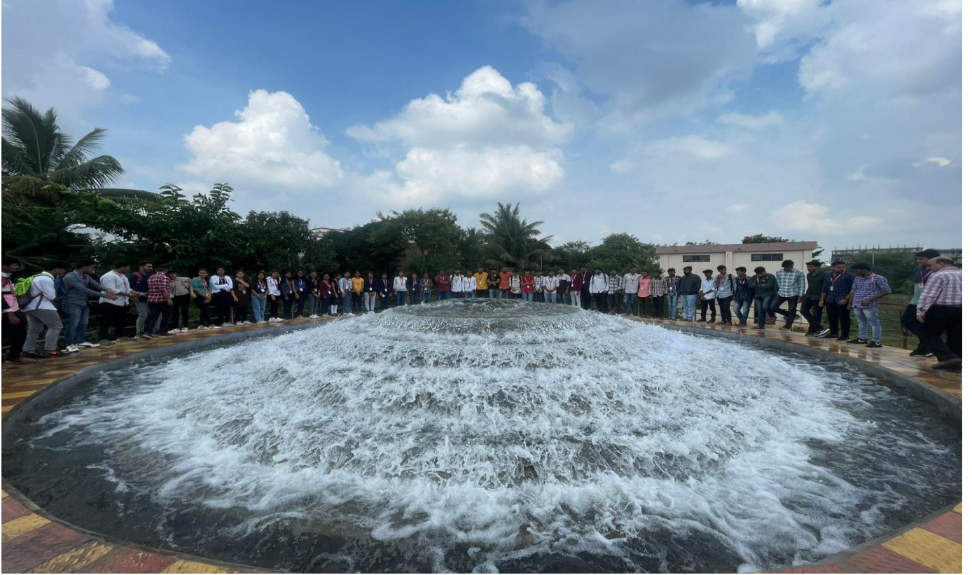
Cascade Aerator View at WTP
